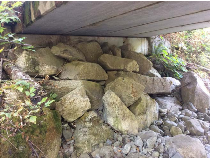
Left Bank Abutment when facing downstream
