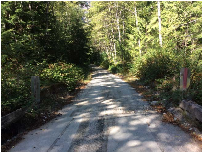
Right approach viewed from bridge
