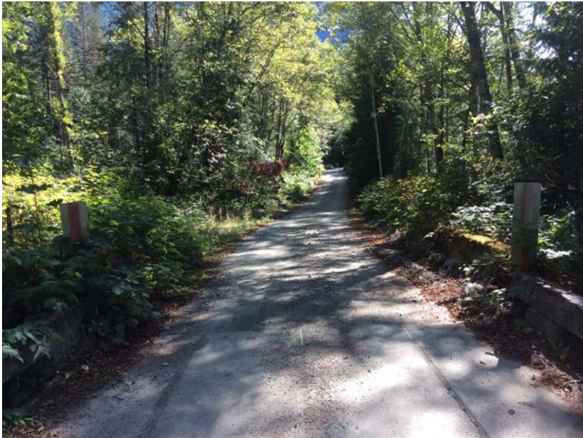
Left approach viewed from bridge
