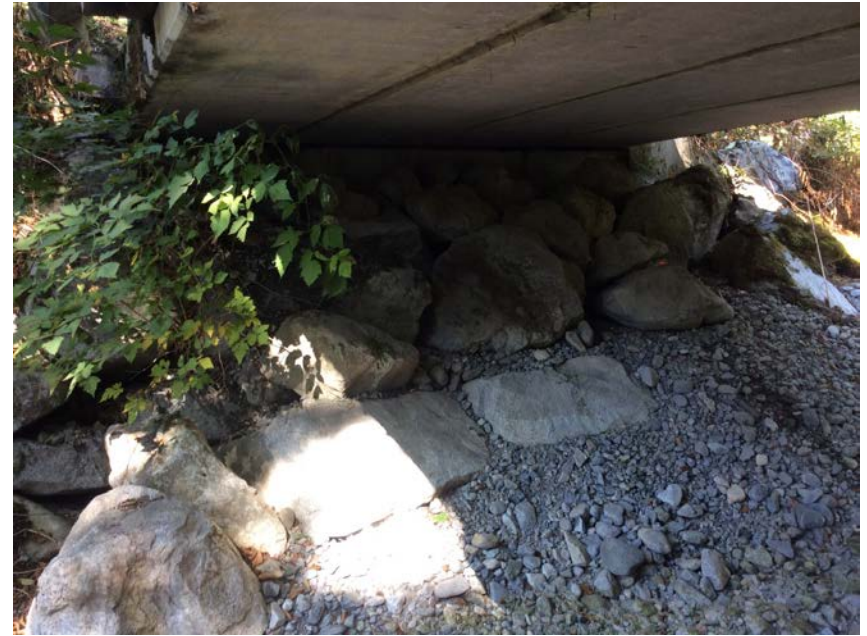
Right Bank Abutment when facing downstream
